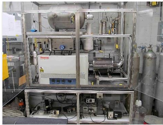
Figure 3.64: Supercritical Water Chemistry and Materials Test Loop
