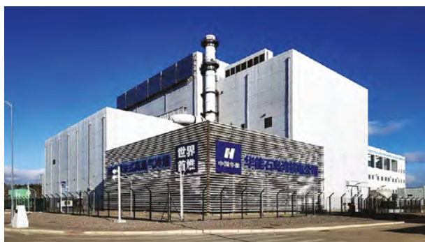
Figure VHTR-1: The nuclear island of the High-Temperature Gas-Cooled Reactor - Pebble-bed Module (HTR-PM), China
