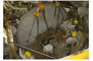
Remove Radiation Shielding Plate
