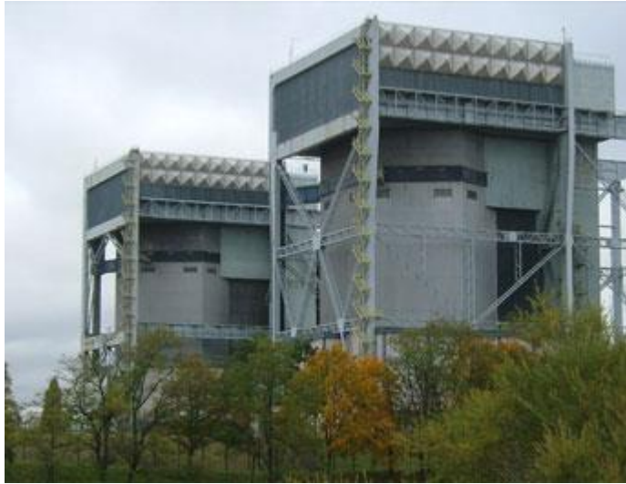
EDF Uranium Naturel Graphite Gaz (UNGG) reactor – Saint-Laurent-des-Eaux (© IRSN)
