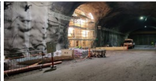
Technical rooms –437 m
