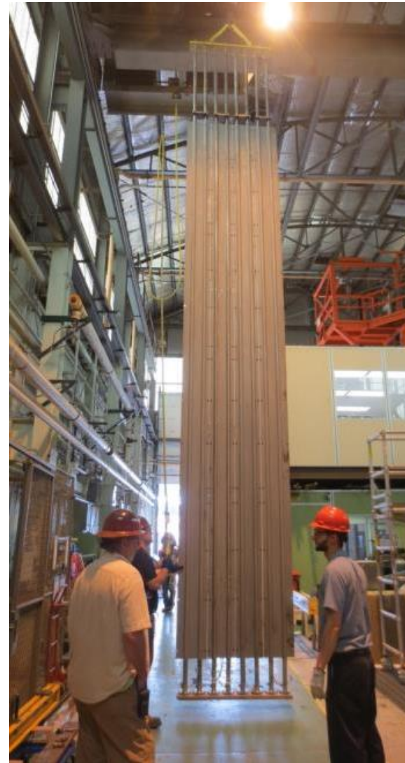
Panel hoisted vertical prior to install
