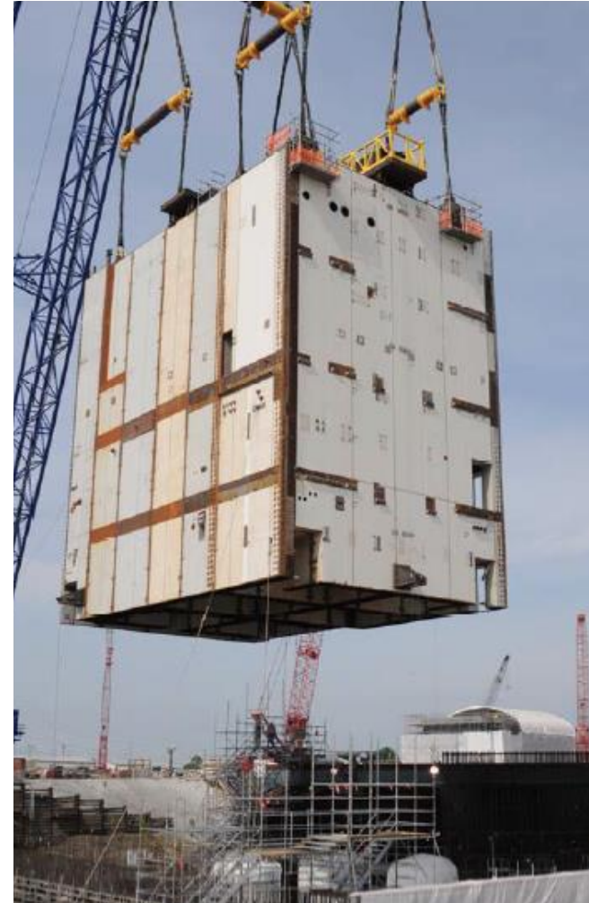
CA20 being set in place by heavy crane
