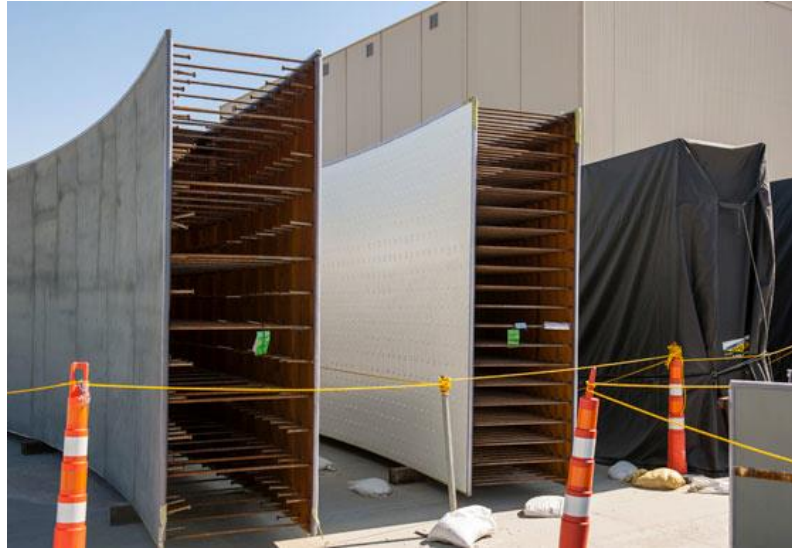
Vogtle Unit 3 shield building wall panels, May 2014
