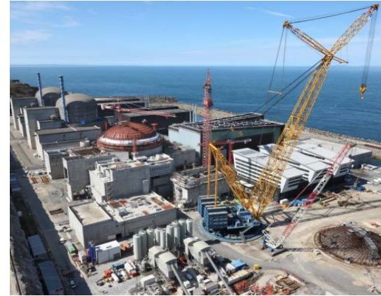
EPR Flamanville Construction site
