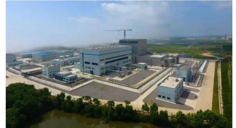
Construction site of HTR-PM
